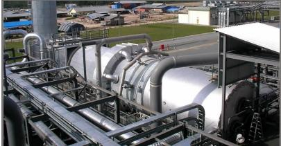
Gas Processing Thermal Oxidizers
